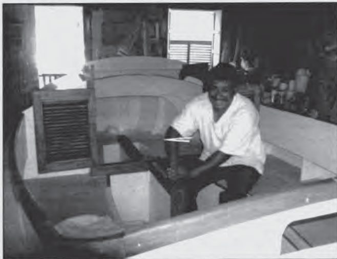
"Chico" doing some finish work.
