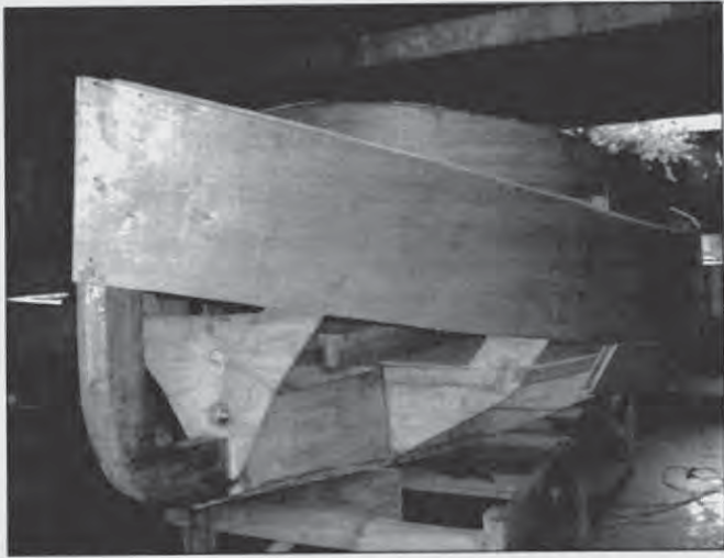
Coamings, cabin sides and front top plank hung.
