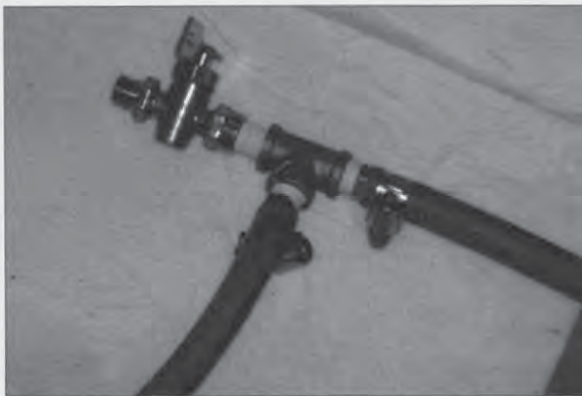
A close-up of the valve assembly on the siphon.
