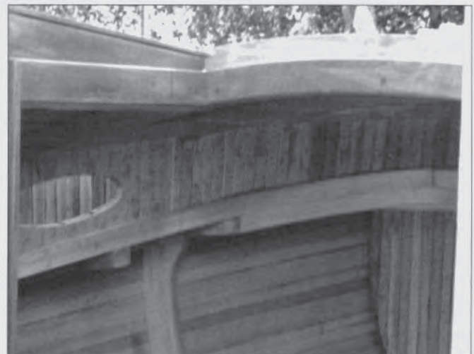
Cabin inside detail.
