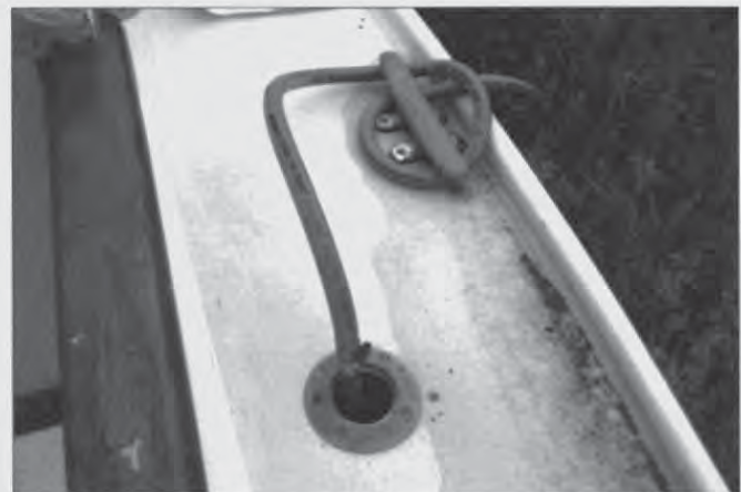
Pipe in tank.
