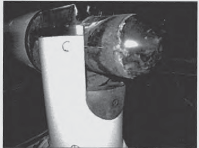
Plug seated where it attaches to mast.
