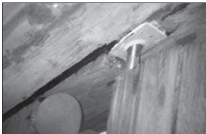
Repaired leak at rudder post.
