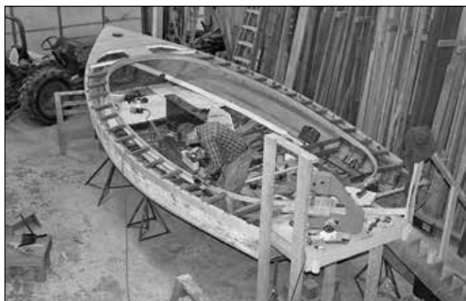
A comprehensive rebuild from bow to stern.
