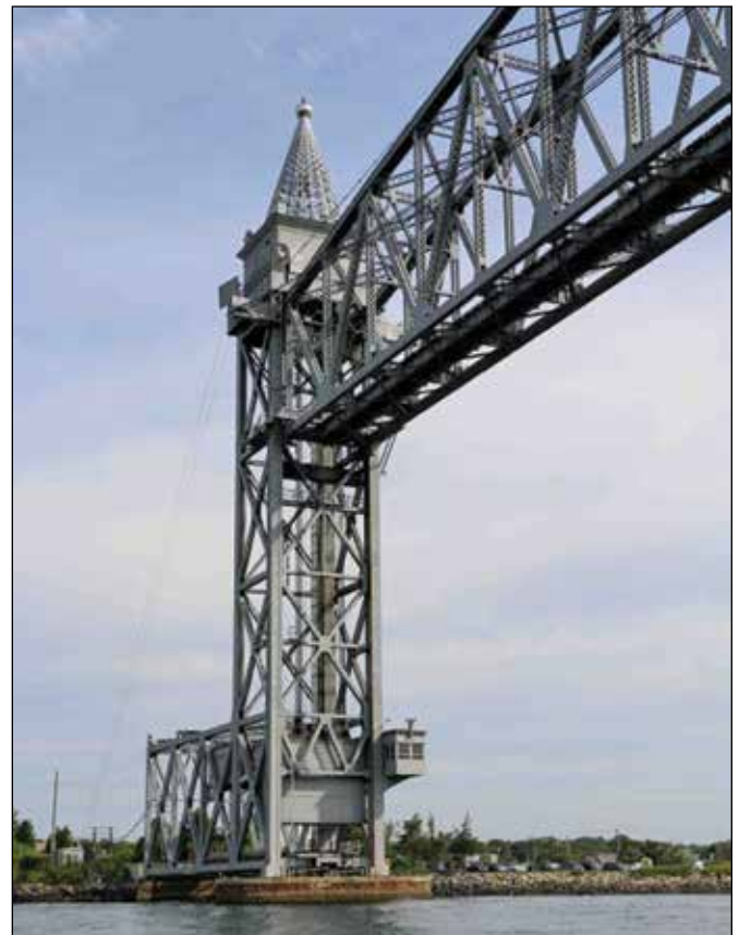
Cape Cod Canal Railroad Bridge.
