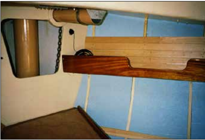
Insulation covered with 2" varnished cedar strips, was applied to the hull and cabin overhead in the forepeak and main cabin.
