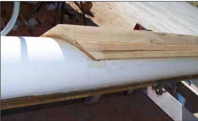
Bottom mast section replaced.
