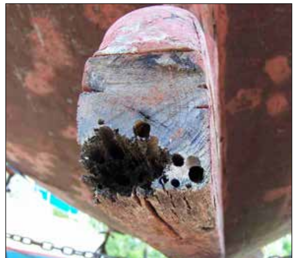
Holes viewable after first cut.
