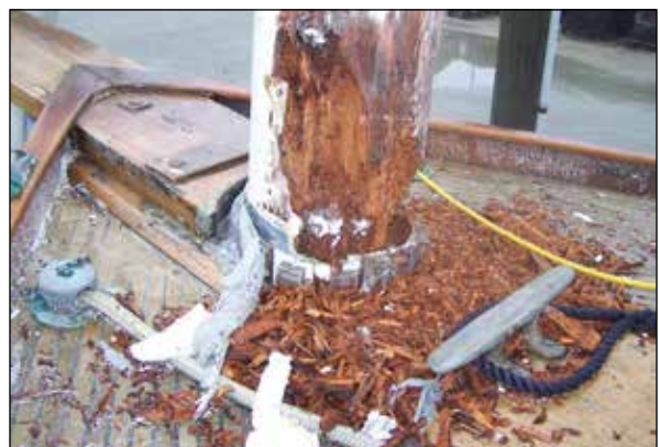
Mast at the deck level.
