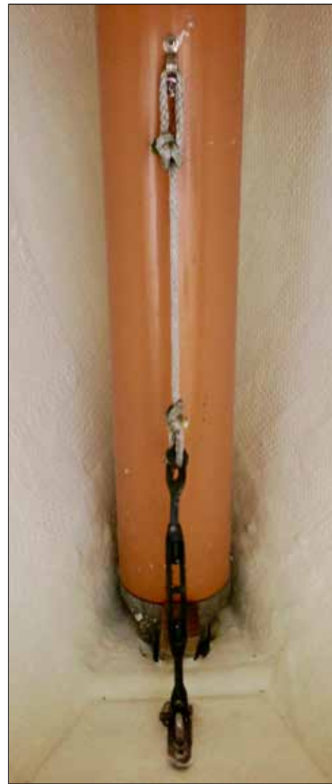
Securing the mast.
