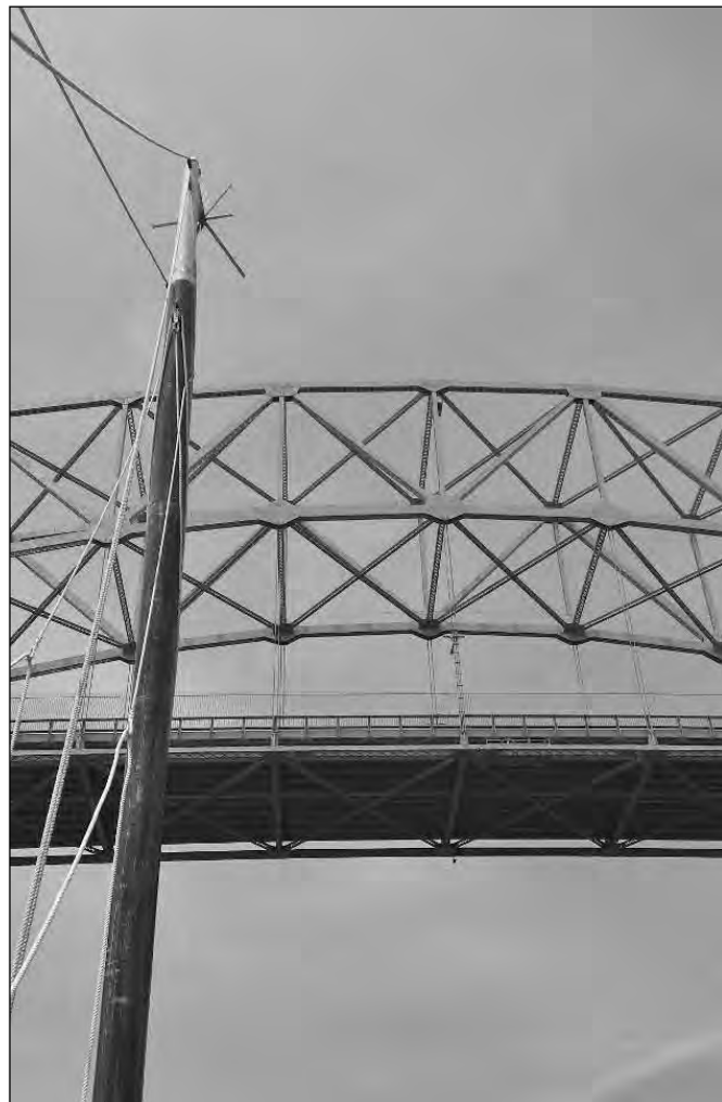
Passing under the Sagamore Bridge.
