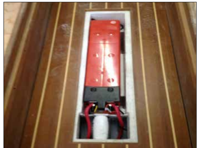
Battery in Keel.
