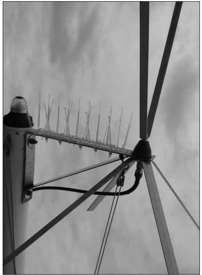
Fig 4 – Bracket Mounted Flat Side Up.
