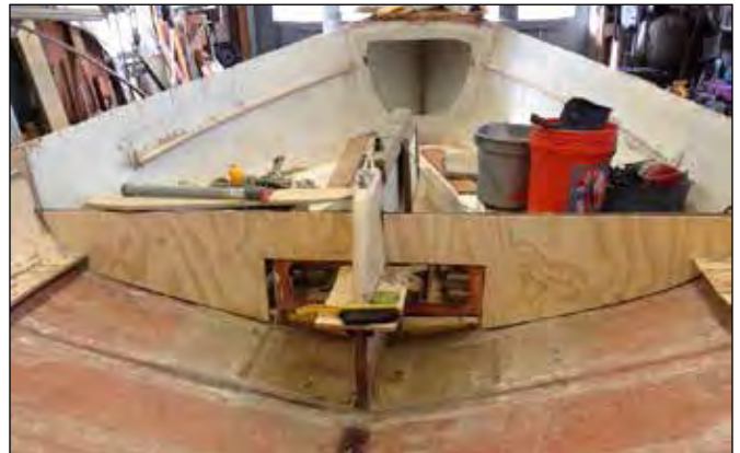
Clean hull; ready for new stringers. Photo courtesy of Judy Sayle.
