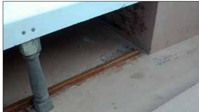
Close up of forward port rail.
