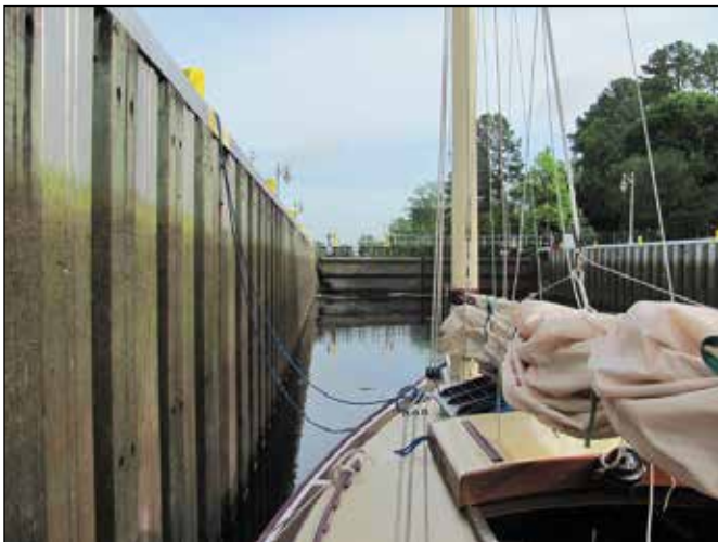
Inside the South Mills Lock.
