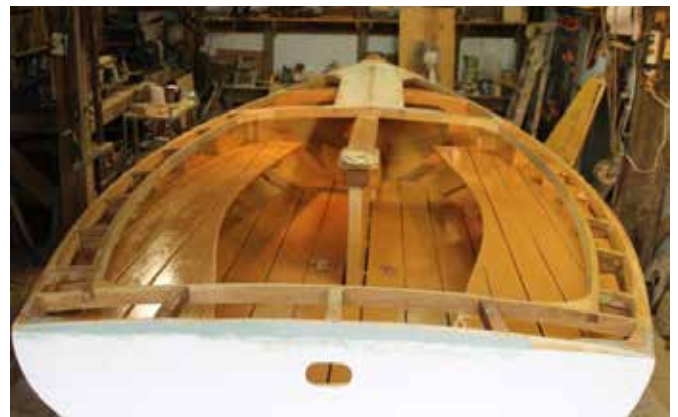
Figure 12. The cockpit flooring and seats installed.
