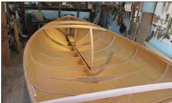
Figure 10. The hull interior all 'glassed in.
