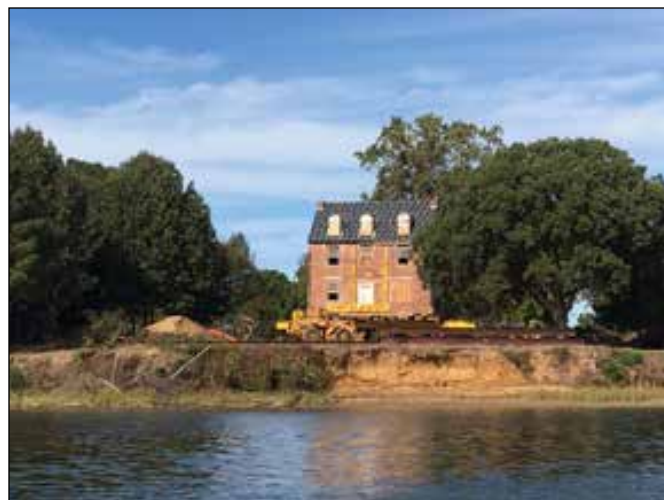
The Galloway House on the Wye.
