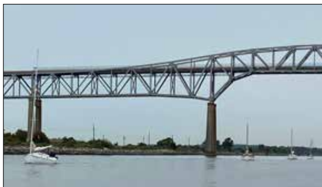
Out of the C&D at Reedy Point.
