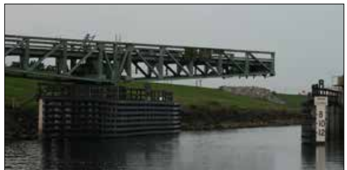
Thomas opening oldest swing bridge in Florida.
