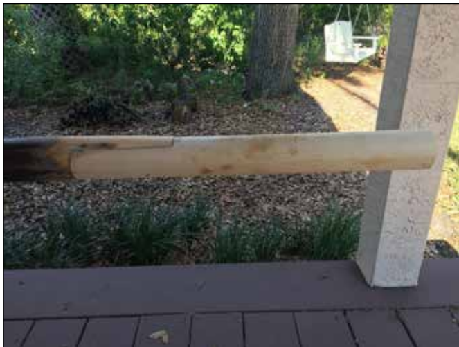
The new section in place.
