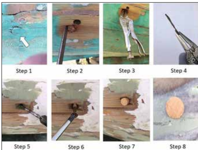
Figure 4. A somewhat unorthodox, eight-step process quickly removes and replaces the offending hardware.
