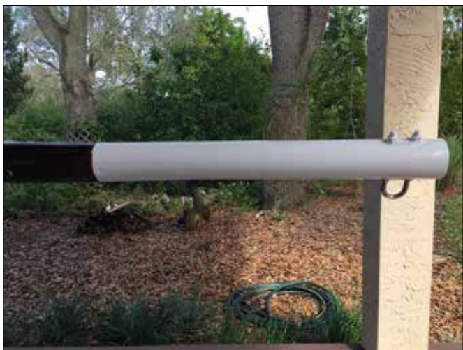
The repaired boom.
