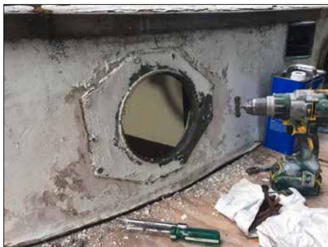
Porthole cleanup underway.
