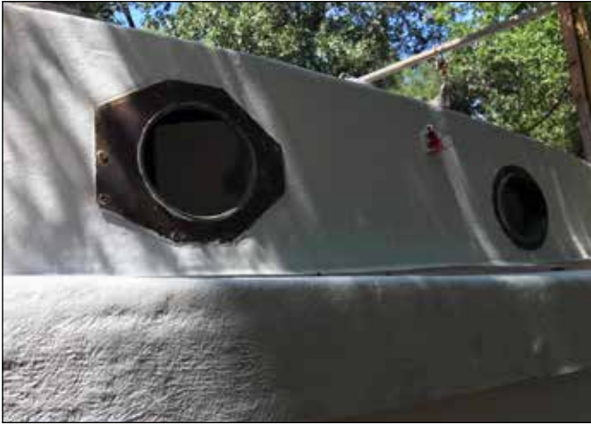
Portholes with excess paint removed.
