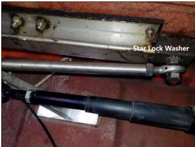
The star lock washer between the steering rod and rack was replaced.
