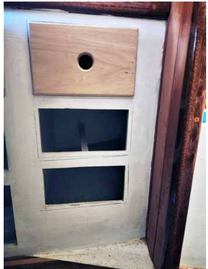
Figure 9. Fitting the test drawer to the openings on the boat.
